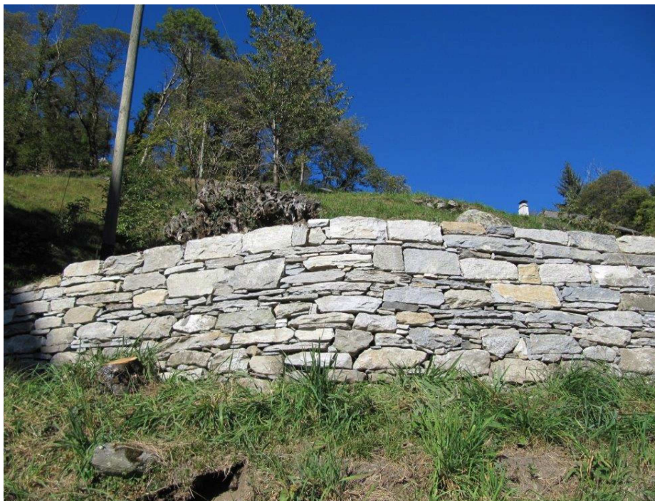
Neue Mauer, Position 6 West
